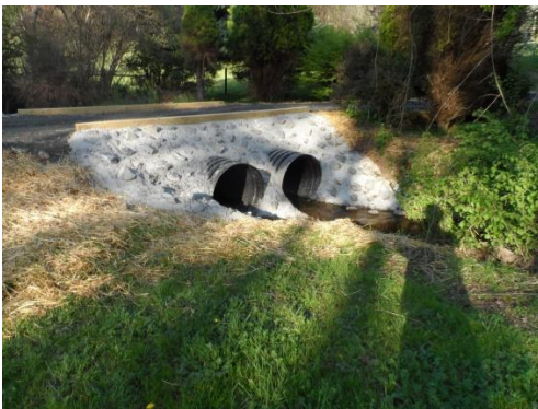
Beaverdam Creek culvert
